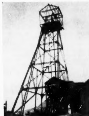
Steel Mine Head Frame
